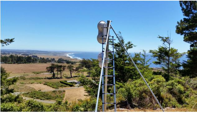
**Figure 1: A hillside relay site with a small mast we built to host multiple long-distance backhaul radios. At this site we host over a dozen backhaul radios and sectors (not pictured).**
